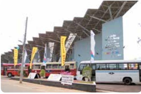
Completed bus terminal with all amenities, Madawachchiya
