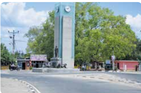
Constructed clock tower - Polonnaruwa branch
