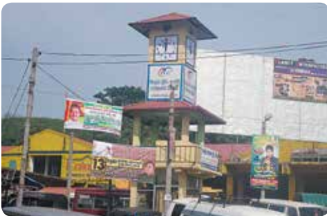
Security watch tower with fixed clock faces - Avissawella branch
